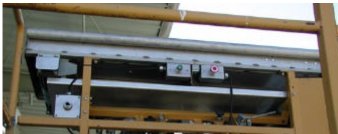
Figure 20: Workstation controls: selector switch (l), momentary pushbutton for semi-automatic function (m), machine emergency stop (r). Difficult to see, but present, are the manual valves for belt conveyor run/stop and the directional valve for the discharge conveyor's swing-out positioning cylinder.
