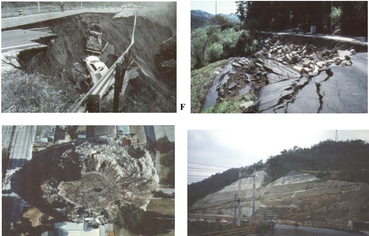
Figure 2-2: Rehabilitation Projects Including: (a) Highway Slope Failure Involving Loss of Life; (b) Roadway Landslide; (c) Sinkhole in Orlando, Florida; and (d) Slope Stabilization.
