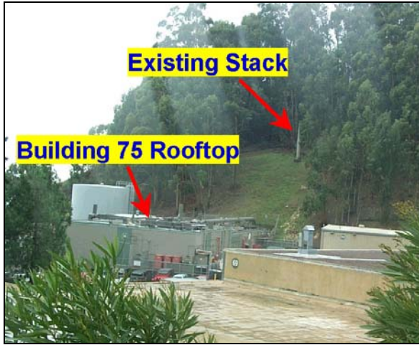
Figure 2: Site Photo of Existing Stack and Proposed Location of Building 75 Stack.
