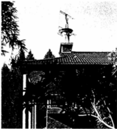
Wind turbine in Zimbabwe.
