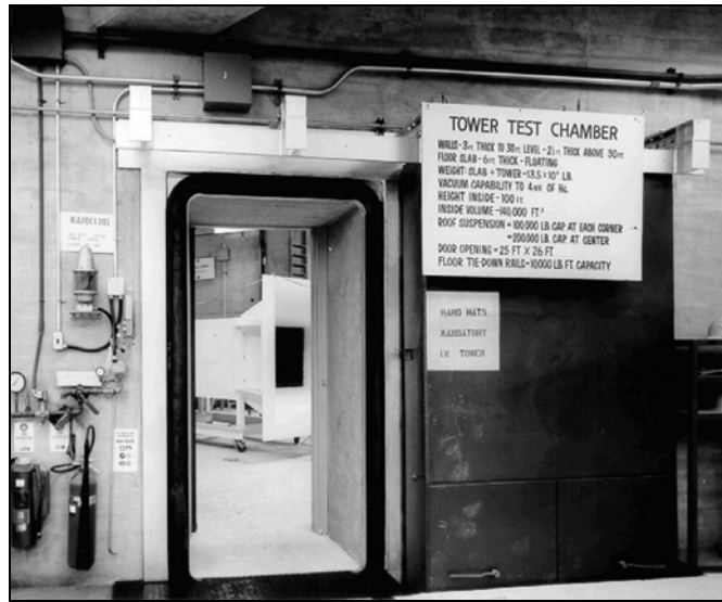
Figure 3.3: View of MARSWIT entrance contraction through the low-pressure chamber access door.
